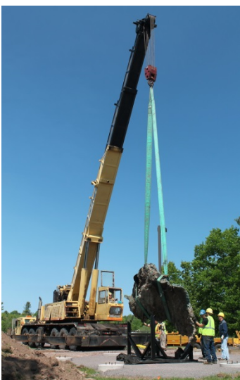
Placing slab on to specially designed stand
