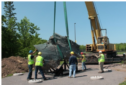
Pushing the slab into position
