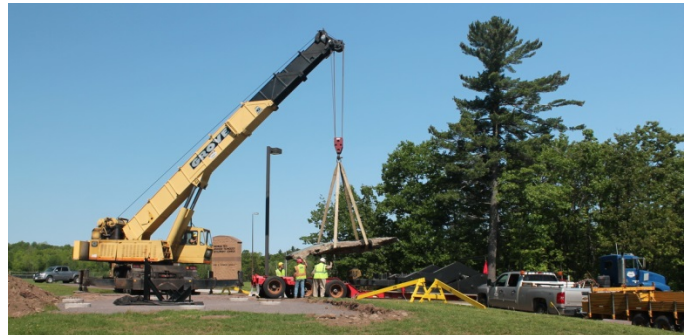
80 ton crane lifting the slab from the trailer
